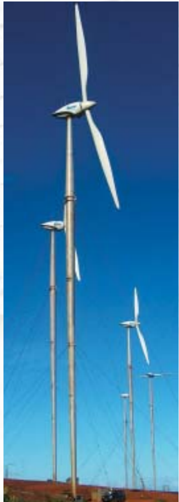
VERGNET WIND TURBINES - KAFEATE (NC)
